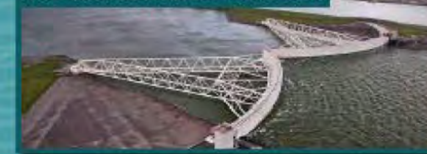
Maeslant Storm Barrier Rotterdam
